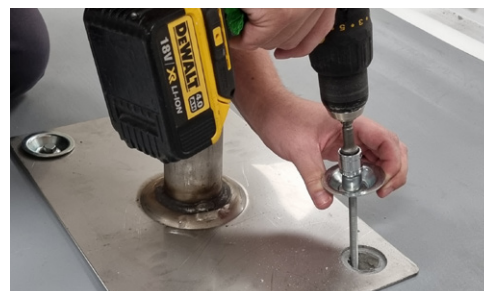
Figure 4 - Correct position of rubber gasket
