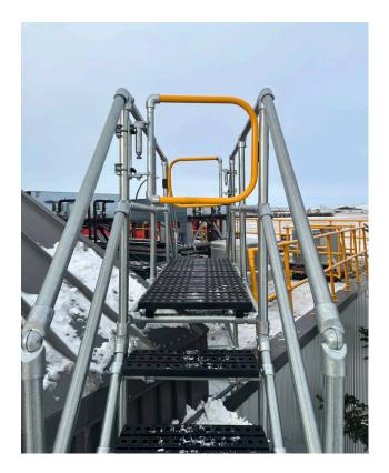
Fixed platforms are ideal for permanent installation. Mobile platforms are equipped with heavyduty locking casters for station-tostation portability that is safer and more efficient than ladders. Work platforms can also be customized for adjustable height, outfitted with racks and shelves, provided with shop services (e.g., air, water, electrical), and furnished with a Kee Gate selfclosing gate.
