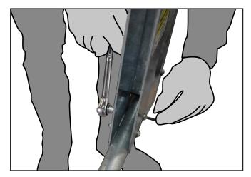
**F.** To extend the gates width to the required opening simply loosen the hex nuts and bolts on the bottom guardrail using a 3/16" Allen Key and  $\frac{1}{2}$ " socket.
