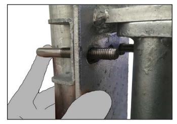
**A.** Align the fixing plate on internal face of the opening, so that the rails of the Safety Gate match up with the top of the Guardrail System. Select the correct U Bolt & pass it through the Steel Safety Clamp, around the support leg/structure and feed through the top holes of the fixing plate.
