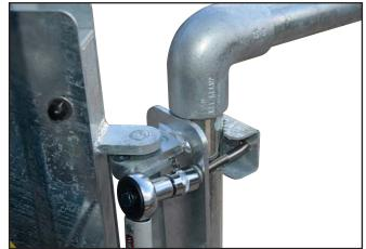
**D.** Torque all nuts/U Bolts to 25Nm using the 11/16" or  $\frac{1}{2}$ " socket and torque wrench.
