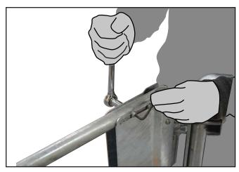
**I.** Once the gate is lined and levelled tighten the hex nuts and bolts on the top & bottom guardrails using a 3/16" Allen Key and 42" socket.
