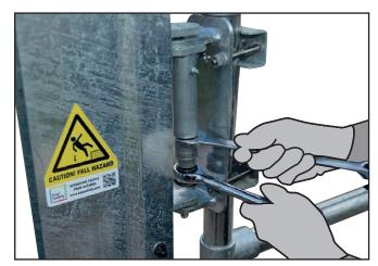
**L.** Using the 15/16" socket & ring spanner start to tighten the bolt until the gate completely closes. (Note:- You may have to hold the socket whilst using the ratchet).
