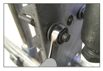
**C.** Select the correct U Bolt & pass it through the Steel Safety Clamp, around the support leg/structure and feed through the middle holes of the fixing plate. Using a  $\frac{1}{2}$ " or  $\frac{11}{16}$ " flat washer and nut connect the U bolt to the Support Leg/Structure and tighten. Repeat step for lower holes in faceplate.
