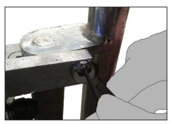
**M.** Using a 3/8" spanner and 3/16" hex key, slacken off the locking nut and adjust the grub screws so that the gate leaves meet in the middle. Once centre position is correct, lock off grub screw using nut.
