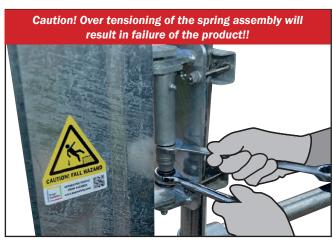
**M.** Once the gate is completely closed tighten the locking nut to hold the tension. Caution:- Continue to hold the ratchet firmly and do not release until the lock nut is tightened. Now remove the socket and spanner from the hinge. Repeat as necessary, to ensure that the gate closes sufficiently, once opened and released.
