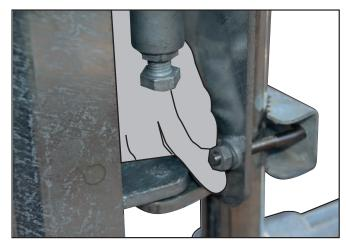
**C.** Select the correct U Bolt & pass it through the Steel Safety Clamp & around the support leg/structure and feed through the top holes of the fixing plate. Using a  $\frac{1}{2}$ " or  $\frac{11}{16}$ " flat washer and nut connect the U bolt to the Support Leg/Structure and tighten.
