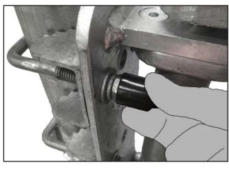
**N.** Ensure all nuts and grub screws (excluding adjustment screw) on the gate are torqued to 39Nm. Finally, place black caps over nuts. Ensure that the structure to which the gate is attached to is sturdy, does not rotate and nuts and grub screws are torqued as per manufacturers guidelines.
