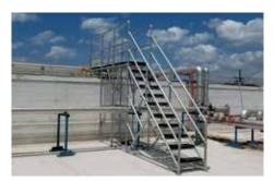
Kee Safety Step-Overs provide a safe route over objects and obstructions on the rooftop. Accommodates metal profile, standing seam and other roof styles without penetrating the roof membrane.
