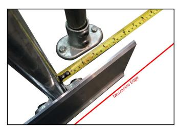
**11.** Check toe-board is central within the frame and tighten nuts to 15Nm to ensure it is held securely in place.
