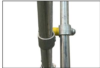
**7.** Ensure frame is parallel. If not, the gate will not operate smoothly. Adjust as necessary by rotating the fittings.
