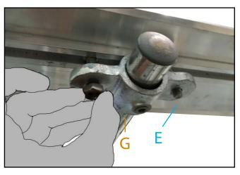
**8.** Mount toe-board (**E**) part to the (**G**) uprights by sliding 4No. bolt heads into the track along the back of the toe-board. Carefully align 2No. bolts so they fit through each of the M51-6 fitting. Add the washer and nut and loosely tighten to permit movement within the toe-board for adjustment in next step.
