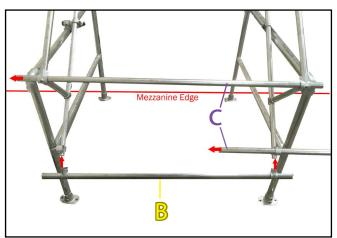
**7.** On opposite end to mezzanine edge add 2no. part ( $\mathbf{C}$ ) horizontal tubes to upper and lower cantilever tubes. Then add part ( $\mathbf{B}$ ) onto ends of lower cantilever tubes. Tighten using 1/4" hex key.
