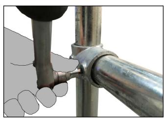
**13.** Ensure all fittings are correctly torqued to 39Nm and all tubes are level. Ensure gate operates smoothly and opens and closes positively.
