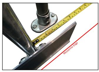
**13.** Check part (**H**) toe-board is central within the frame and tighten nuts to 15Nm to ensure it is held securely in place.
