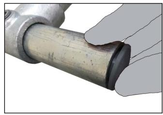
**14.** Place plastic end caps on all exposed tube ends. These may need to be tapped into place using a rubber mallet.
