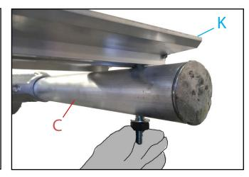
**11.** Add 1no. part ( $\mathbf{K}$ ) toe- board to part ( $\mathbf{C}$ ) uprights. Thread M10 x 80mm bolt through hole in upright and add nut and washer. Tighten to 15Nm.
