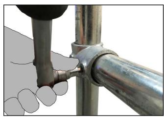
**14.** Ensure all fittings are correctly torqued to 39Nm and all tubes are level. Ensure gate operates smoothly and is balanced.
