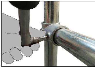
**10.** Ensure all fittings are correctly torqued to 39Nm and all tubes are level. Ensure gate operates smoothly and opens and closes positively.
