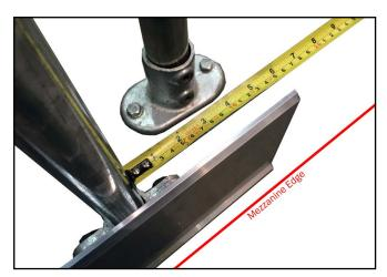
**9.** Check toe-board is central within the frame and tighten nuts to 15Nm to ensure it is held securely in place.
