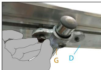
**10.** Mount toe-board (**D**) part to the I uprights by sliding 4No. bolt heads into the track along the back of the toe-board. Carefully align 2No bolts so they fit through each of the M51-6 fitting. Add the washer and nut and loosely tighten to permit movement within the toe-board for adjustment in next step.
