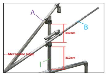
**6.** Carefully measure and mark 310mm from top of frame as shown above. Slide part  $(\mathbf{B})$  onto part  $(\mathbf{I})$  and mount fitting at this mark, ensuring bearing is on the inside of the frame then tighten grub screw. Measure and mark 240mm from top of fitting on part  $(\mathbf{B})$ . Add part  $(\mathbf{A})$  to part  $(\mathbf{I})$  mouting the fitting to this mark ensuring bearing is facing same direction and tighten grub screw. Repeat process for other frame.
