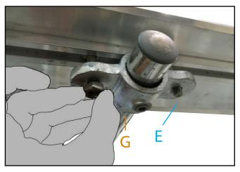
**8.** Mount toe-board (**E**) part to the (**G**) uprights by sliding 4No. bolt heads into the track along the back of the toe-board. Carefully align 2No. bolts so they fit through each of the M51-6 fitting. Add the washer and nut and loosely tighten to permit movement within the toe-board for adjustment in next step.
