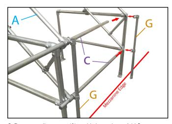
6. Rotate cantilever part (A) so this is as above. Add 2no. part
