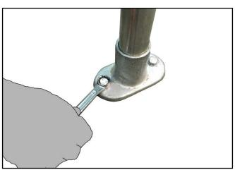
**4.** Using the 4No (62-8) castings at the base of the frame legs mount all 4No. feet to the floor. Ensure fixings are torqued as per suppliers' guidelines.
