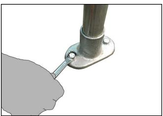
**4.** Using the 4No (62-8) castings at the base of the frame legs mount all 4No. feet to the floor. Ensure fixings are torqued as per suppliers' guidelines.
